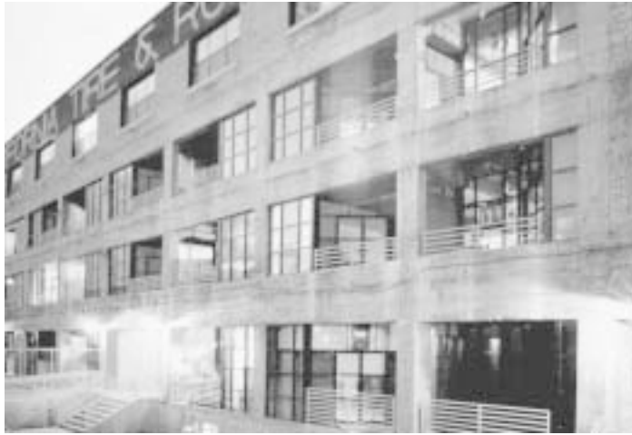
Rehabilitation of an industrial building in Salt Lake City for live/work lofts. The original concrete building material remains exposed contributing to the projects unique appeal and retaining its identity. The original window openings have also been retained and modified to suit the new use.
